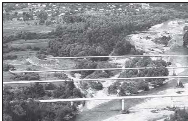
Fig. 8.17: Pipelines transporting natural gas in Ukraine
